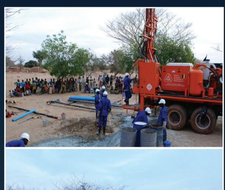
To date the rig has drilled 429 boreholes with a total meterage of 34,790 and a success rate of 73% and as a result 148,200 people in the country are benefiting from access to clean water.
