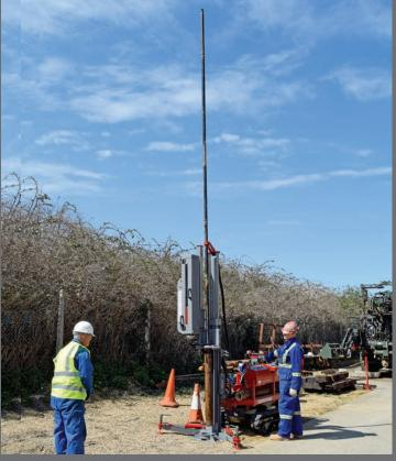
height allowing easier tool handling and installation Drill string is supported by a stainless steel rod guide.
